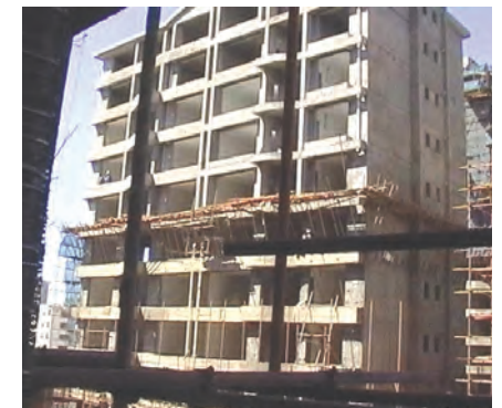
Earthquake resistant building made with COFFOR ® shear walls
