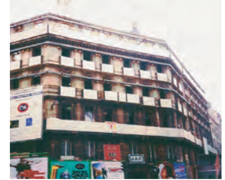
Renovation of a historical 8-story building
