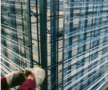
Easy rebar insertion
