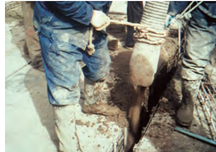
Concreting with a pump
