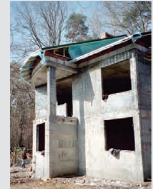
Villa in construction
