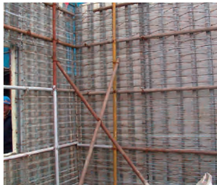
Light bracing (steel tubes) with COFFOR®
