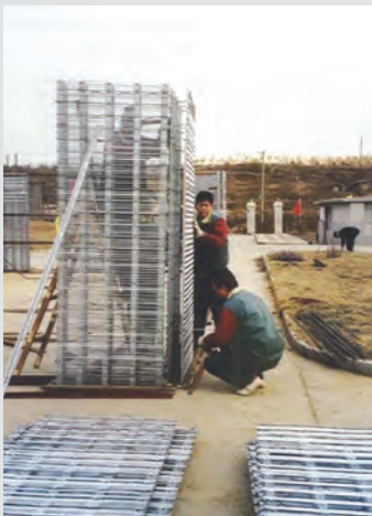
Unskilled worker trained on-site
