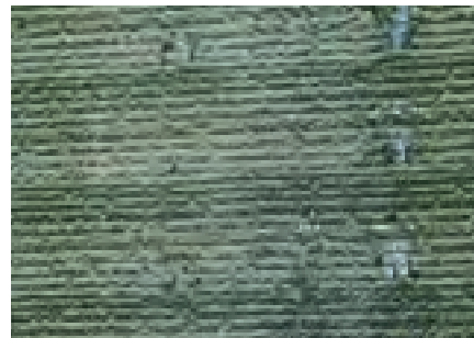
Close view of COFFOR ® after concreting
