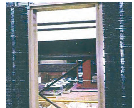
Edge closing with wood planks
